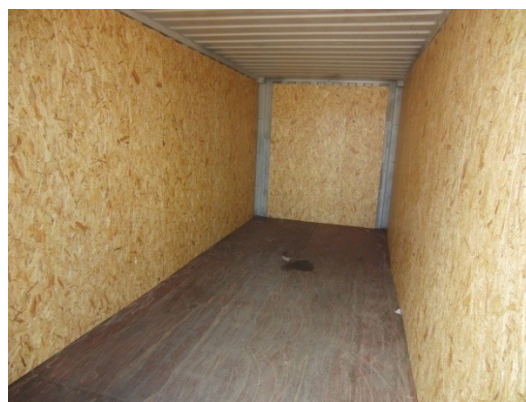
Figure 7.53 Lining a 40-foot container with chipboard panels
