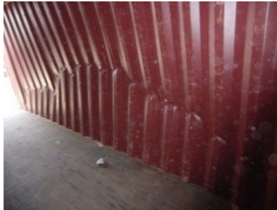
Figure 7.50 Damaged CTU side wall
