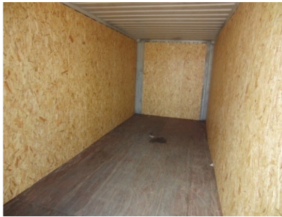
Figure 7.53 Lining a 40-foot container with chipboard panels
